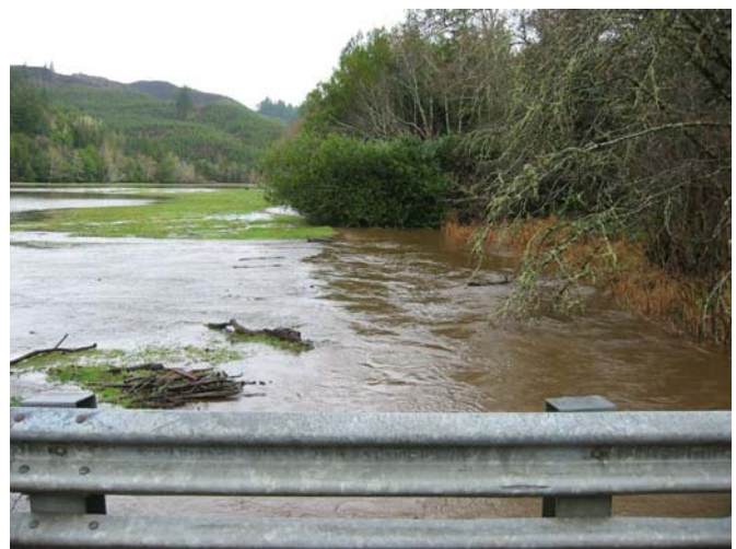
Figure 3.6. Big Creek overflows
