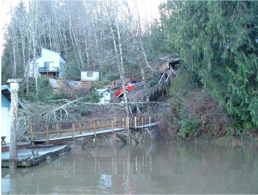
Figure 4.6. Catastrophic failure of slope and septic system.
